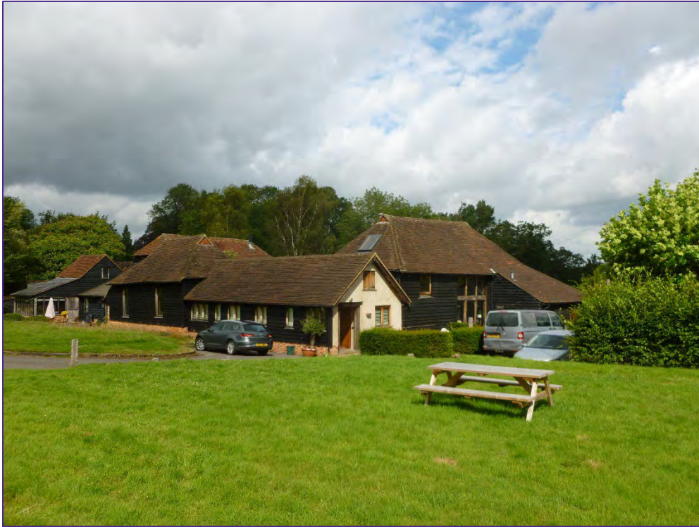
Plate 16: The Brew barn with later additions viewed north-west from private grounds of barn.
