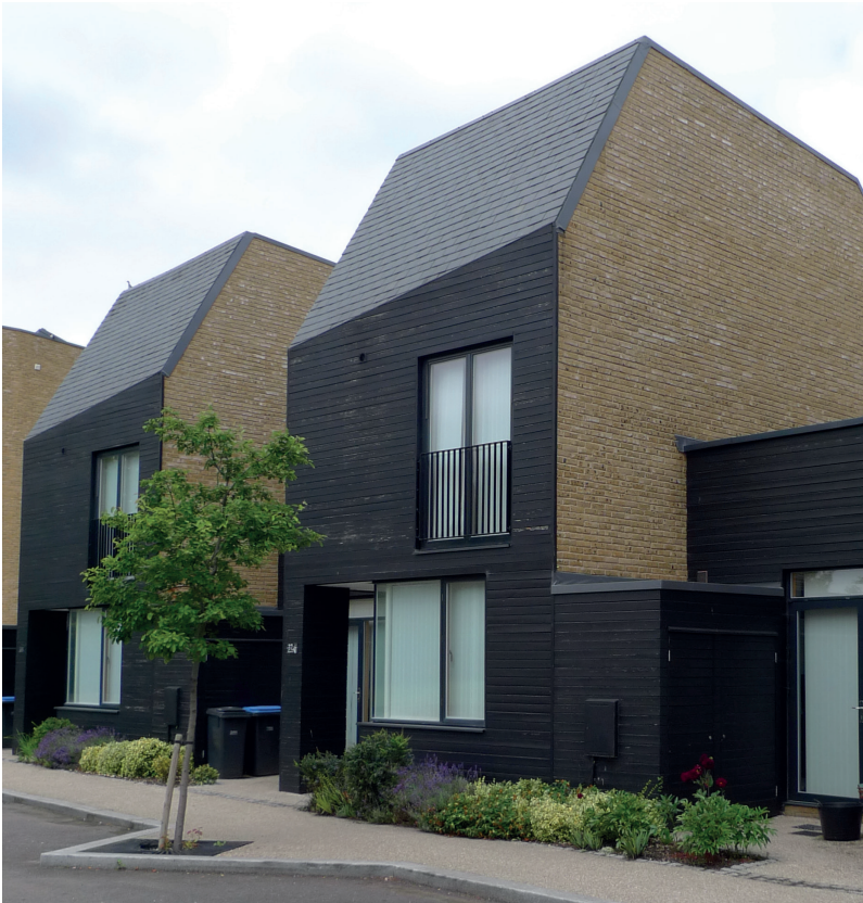
A simple palette of materials can create a coherent sense of place but all materials need to be robust and able to withstand weathering. An example of timber cladding that has started to show signs of wear at Newhall Be by Alison Brook Architects. Photo credit: Allies and Morrison.
