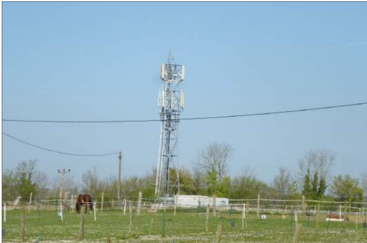
View North from footpath
